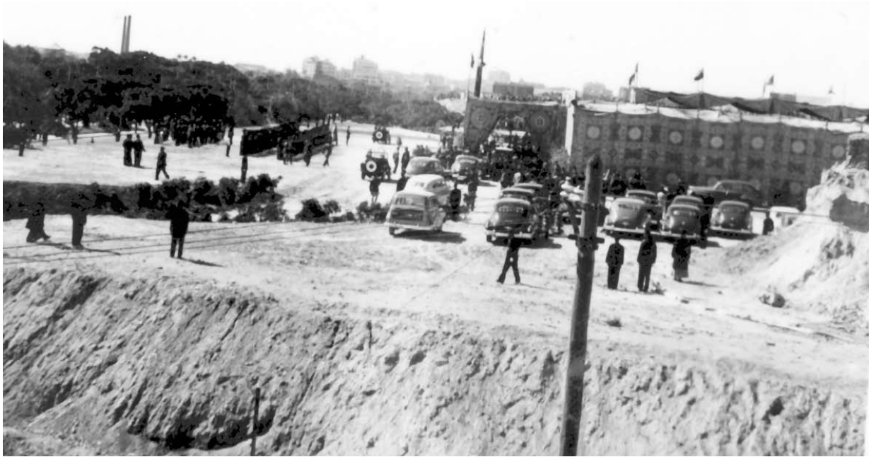
The site where the Faculty of Engineering of the University of Alexandria was to be built. This photo was taken by my father from the balcony of our house on the day of the laying of the foundation stone by King Farouk in March 1950.
